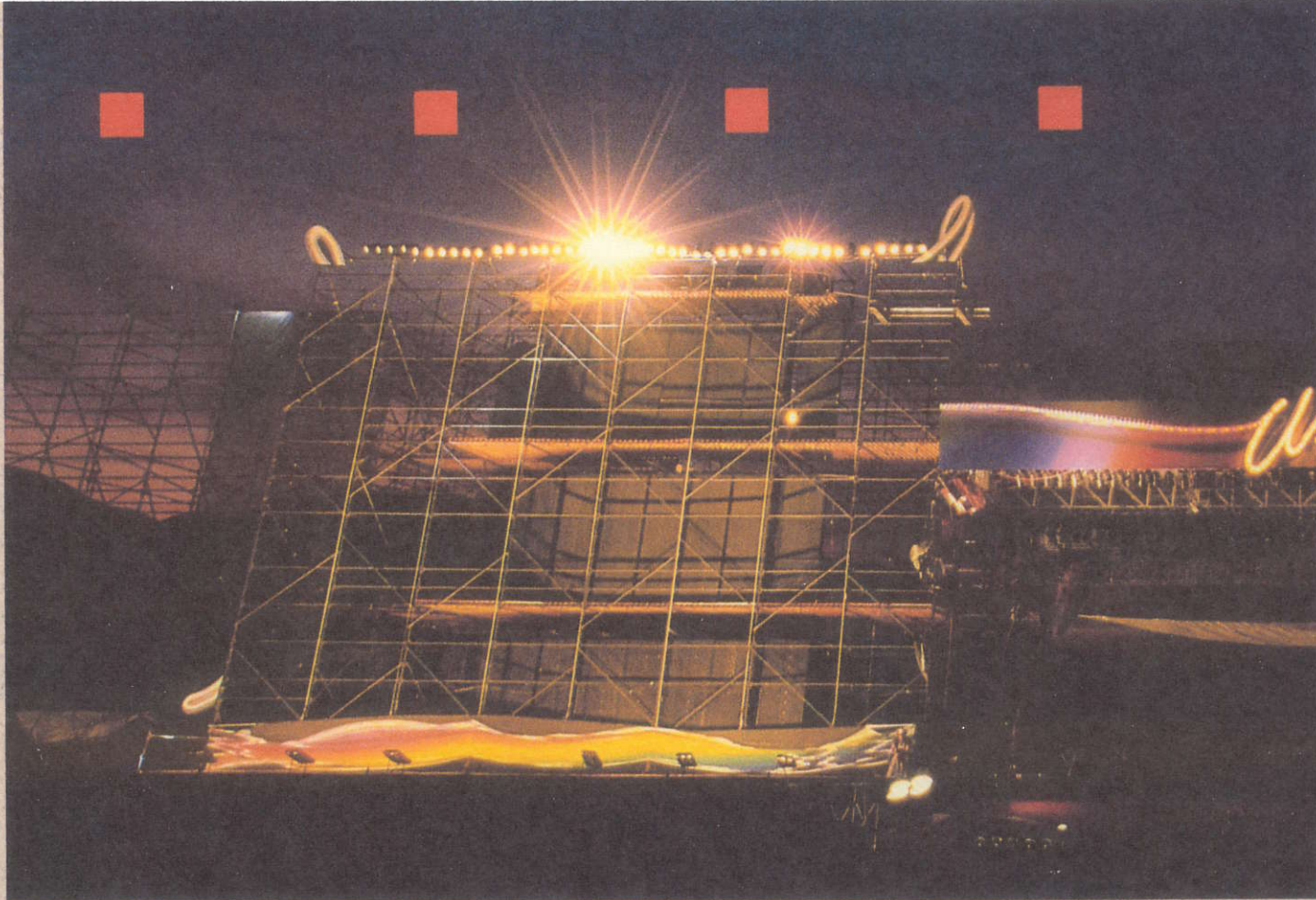
More than 2,400 individual loudspeaker components made up the 400,000 Watt JBL sound system built to power the three-day "US Festival" in Southern California.
